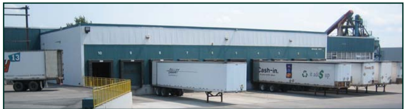
Renovations to the ABCRC loading doors at the Calgary Plant have reduced live loading time.
