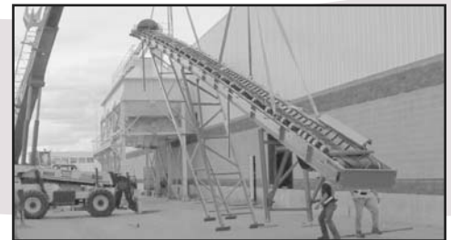
Conveyor installation at Edmonton Plant
